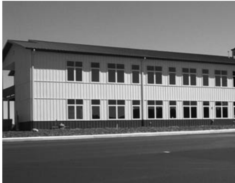
Organic Valley's 49,210 square-foot "green design" headquarters in LaFarge, WI.
