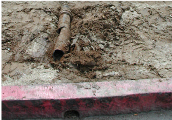
Old rainwater downspout outlet
