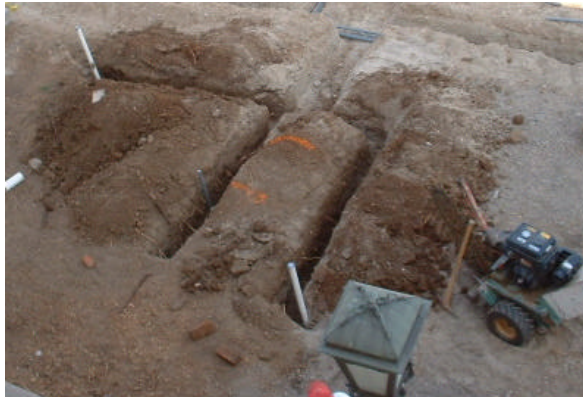
New irrigation and drain lines
