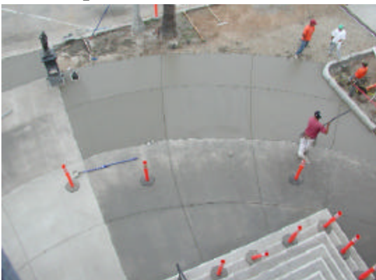
New pavement areas
