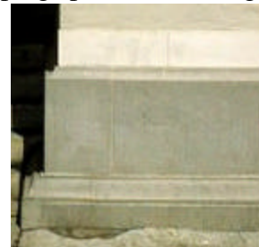
...and after cleaning.
