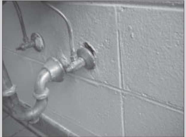
This escutcheon plate is loose. All possible pest entries should be patched, sealed or closed.
