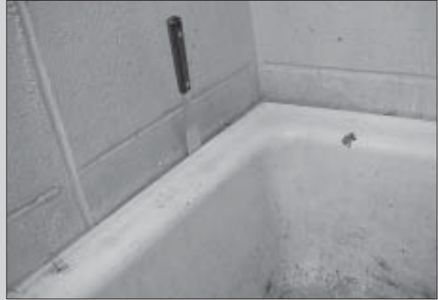
An icing spatula shows that the seal around a sink is missing, identifying the space that pests use to move around.
