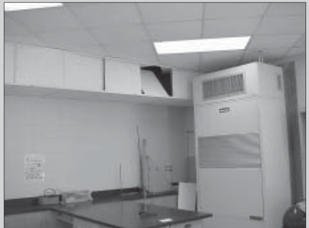
Replace missing or damaged ceiling tiles.
