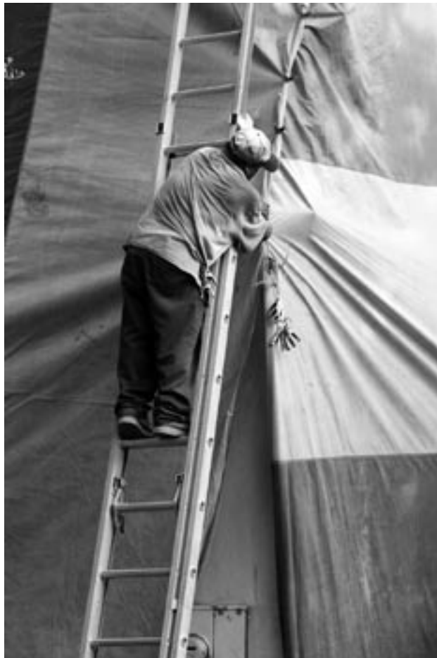
A laborer tents a house for Vikane fumigation.
